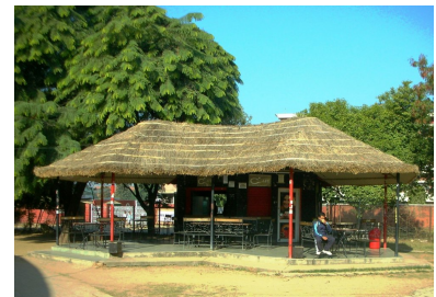
Figure 72: A low-cost cafeteria at Chandigarh Lawn Tennis Association Complex.
