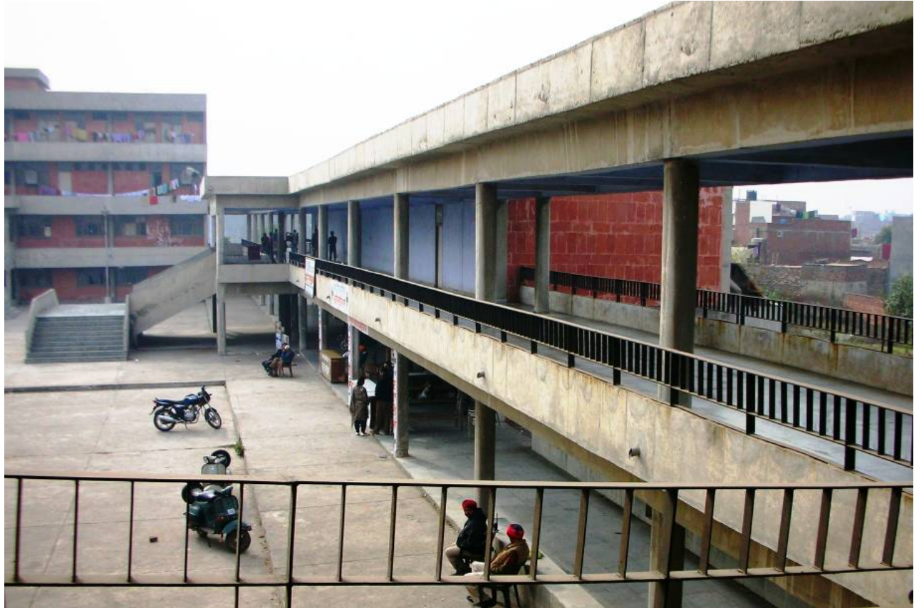
Figure 44: Two-tier link corridor connects shopping arcade/café with voluntary unit and serai building.
