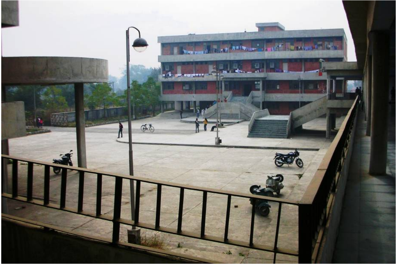
Figure 46: View of court in between cafeteria, serai and voluntary unit.
