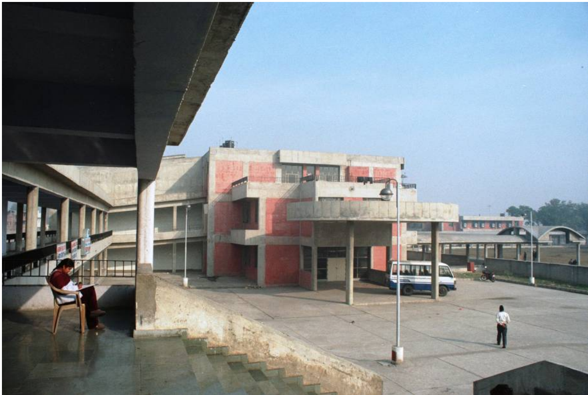
Figure 39: Voluntary unit – view from cafeteria.
