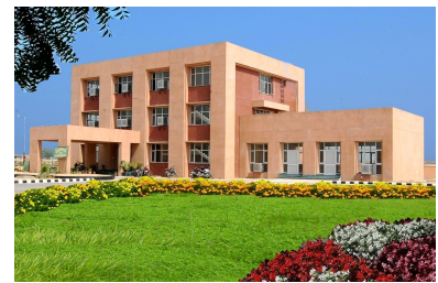
Figure 68: Citrus Estate, Abohar, Punjab. Ducts and storage cupboards, placed along the outer periphery, act as cavity-walls and protect the interiors from external heat.
