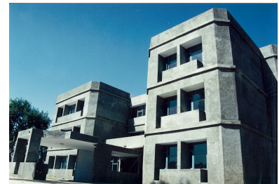
Figure 69: Zila Mandi Bhawan, Fardikot, Punjab. Most of the external surfaces remain in mutually created shade.
