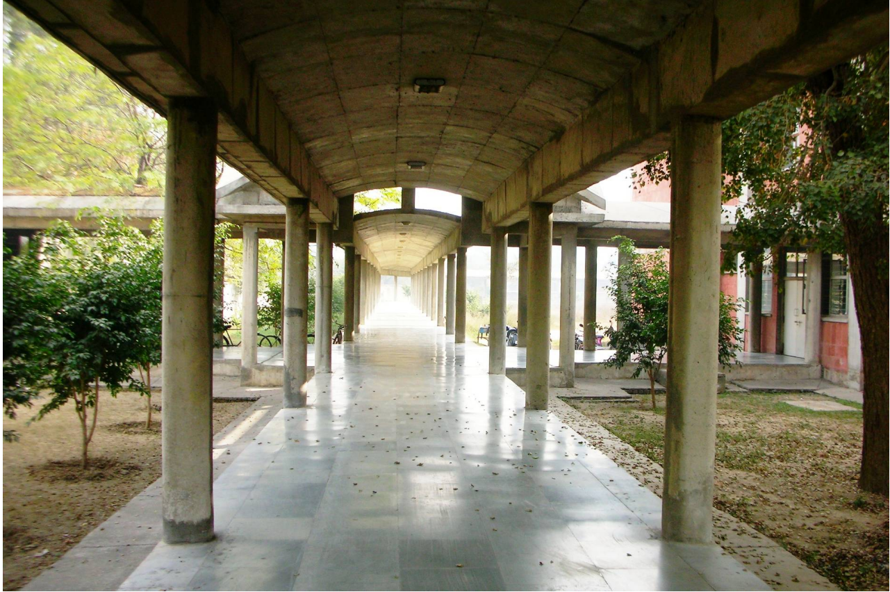
Figure 9: Vaulted corridor runs independently through open spaces
