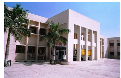
Figure 66: Front facade of Civil Hospital, Samana, Punjab, showing clarity in structural system.
