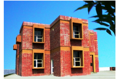
Figure 74: Soil Testing Laboratory, Nawanshahar, Punjab.
