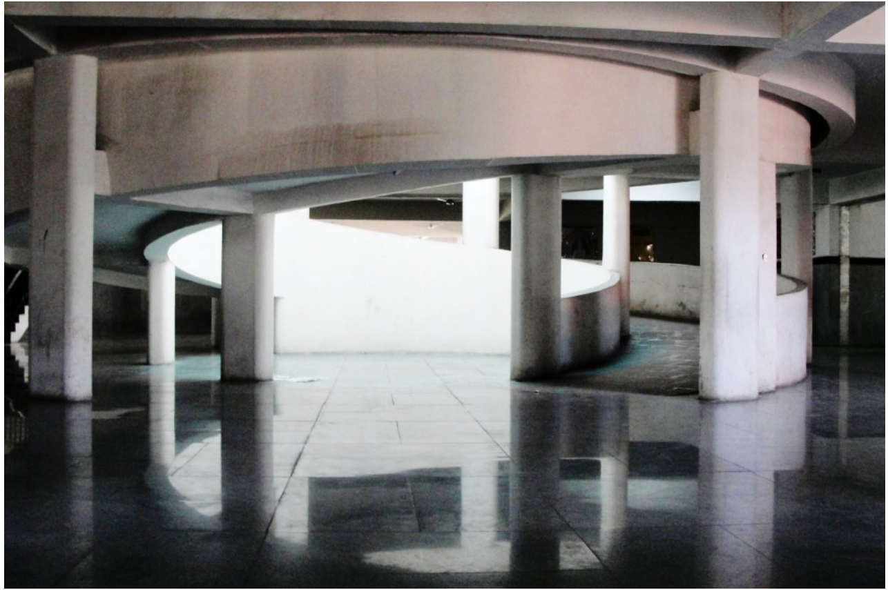
Figure 17: View of ramp in OPD block
