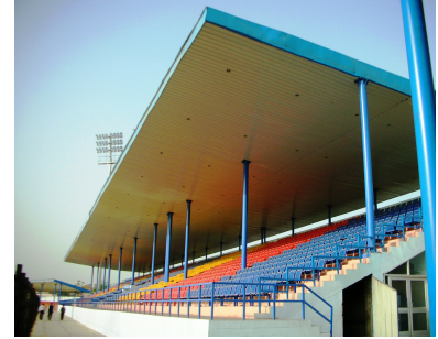
Figure 67: Pre-engineered steel structure of Multipurpose Sports Stadium, Bathinda, Punjab.
